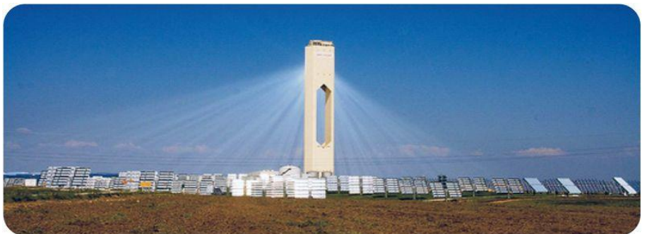
This solar power plant uses mirrors to focus sunlight on the tower in the center. The sunlight heats a liquid inside the tower to a very high temperature, producing energy to make electricity.
